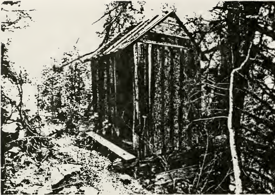
Figure 237. Outhouse located near Structure #126, southwest view.
